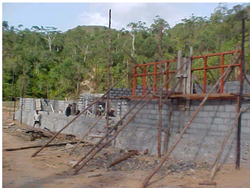
CONSTRUCTION OF EXTERNAL WALLS
