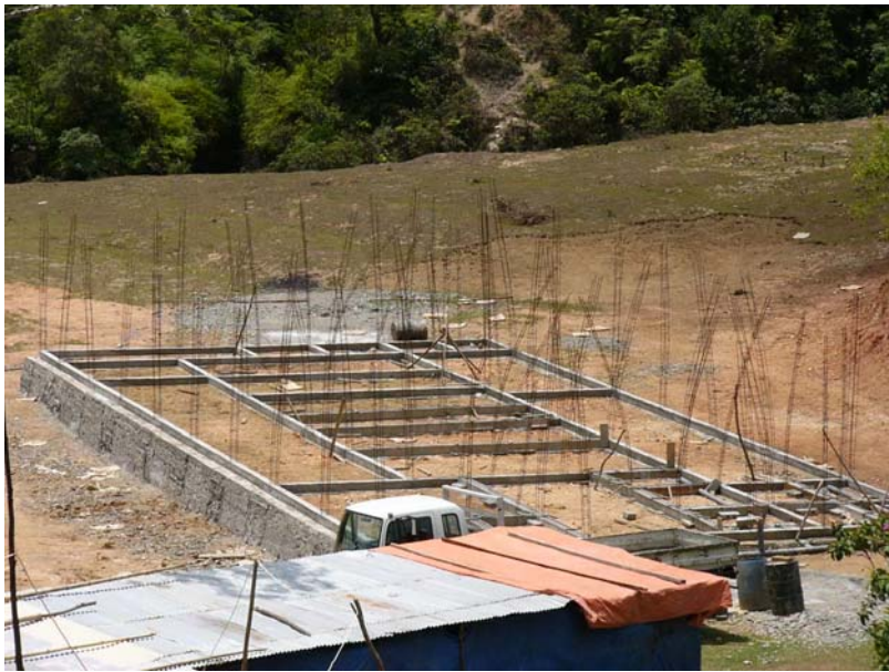
BUILDING FOUNDATION WORK
