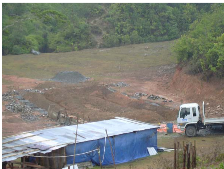
SITE CLEARANCE AND PREPARATION
